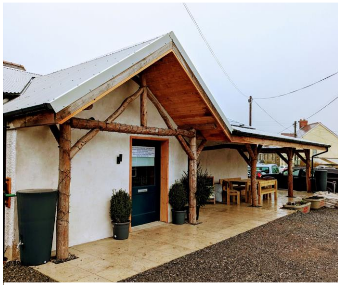
Y Stiwdio eco-building.
